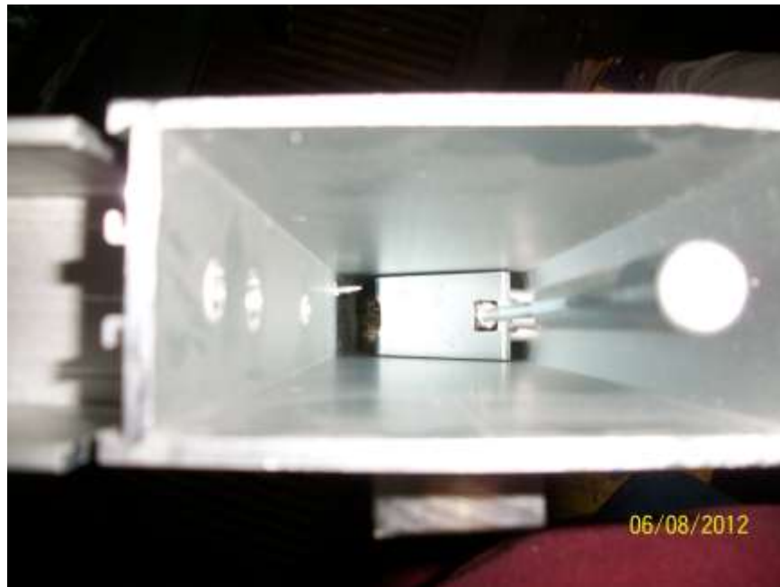
Photo No. 2 Flush Bolt Guide Block Disengaged
